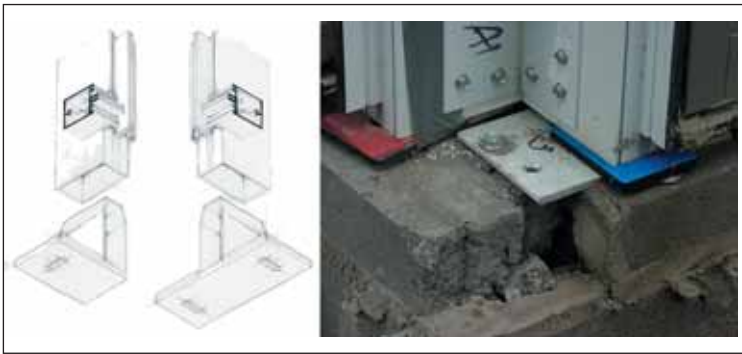
Figure 8. Examples of transom discontinuity.
